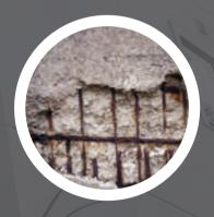
AIR VOIDS AND HONEYCOMBING CAN LEAD TO STRUCTURAL ISSUES AND NON-COMPLIANCE IN FIRE AND ACOUSTICS.
