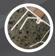
Conventional concrete is porous which leads to corrosion and concrete degradation issues.
