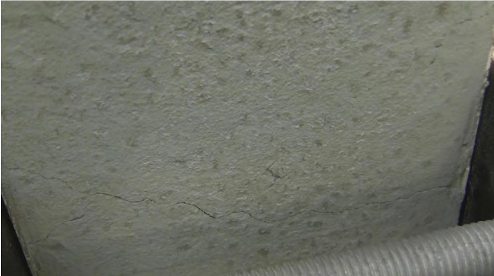
Figure 5.14 (c) Close Up View of Crack at X = 700mm
