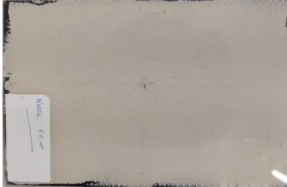
Image 4: No water leakage observed.
