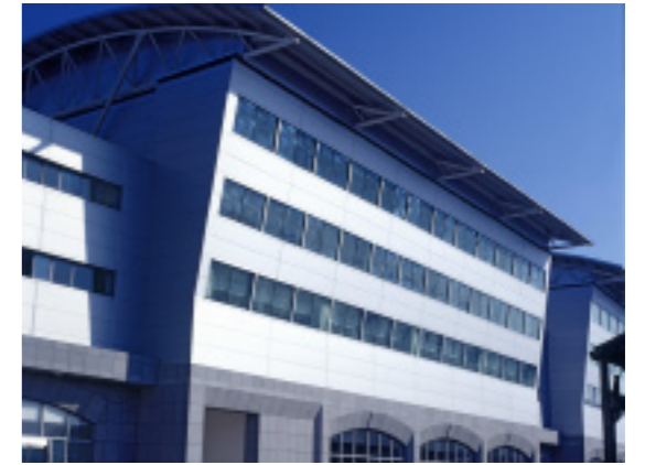
Above : Changchun Railway Station, China Architect: The Third Railway Survey and Design Institute Group Corporation (TSDI for short) Product : Sandwich Wall Panel Facade
