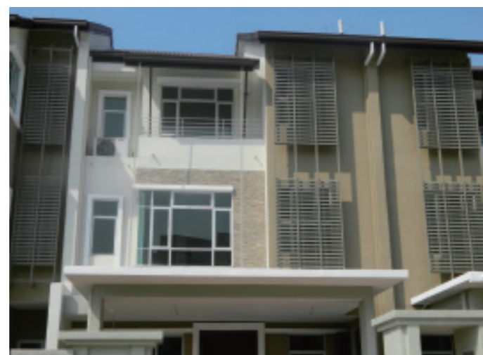
Above : USJ Height Residence, Malaysia Architect: Sime Darby inhouse Product : 70S
