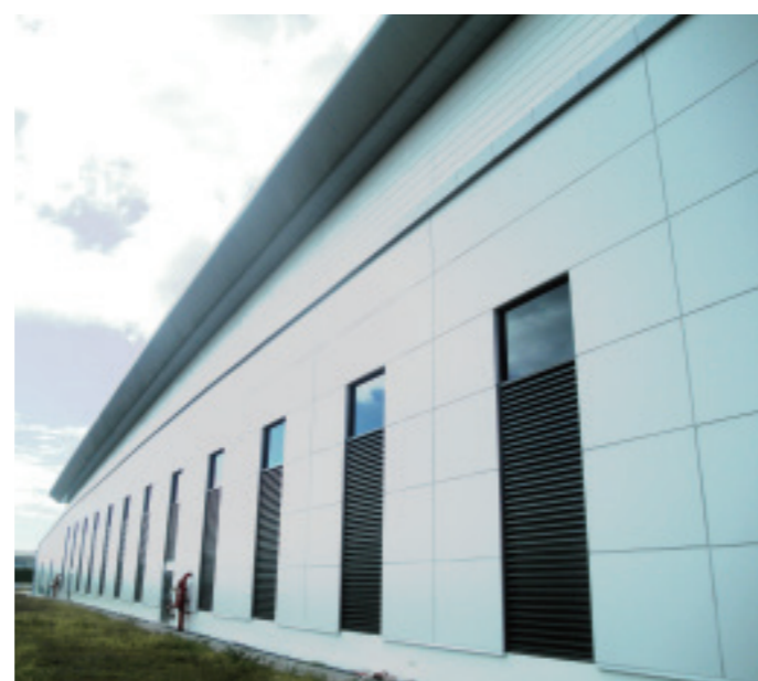
Above : Nestle Warehouse Tanauan Batangas, Philippines Architect: AIDEA Philippines Inc Product : 132S
