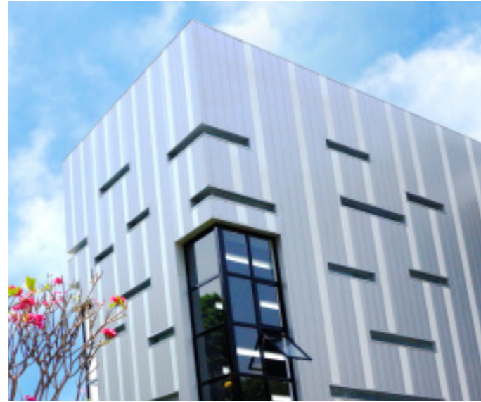
Above : Taman Dayu Residence, Indonesia Architect: Samuel A. Budiono & Associates Product : LinearClad™ F
