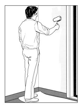
Apply adhesive on the wall area where the first sheet will be installed and a few cm past the seam edge. Apply adhesive in accordance with manufacturer's instructions. You can use a 'lambs' hair' roller but if you prefer to apply the adhesive with a fine-notched trowel, we recommend a TKB A4 model and you can even out the adhesive with a roller.
