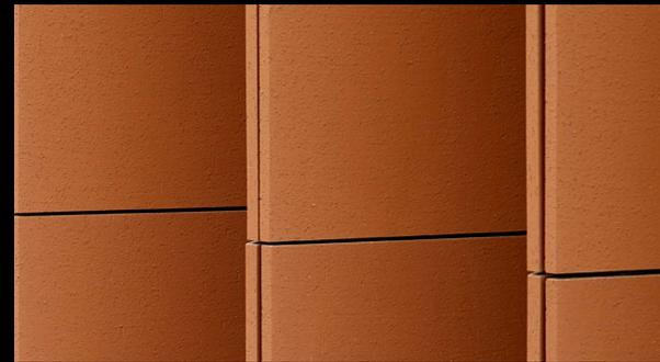
By means of combs, in fine or medium, a profile of long running lines results. The use of chamotte and the removal of the surface lead to a „peeled“ surface whose grooves speak their own language. The grinding of the natural terracotta leads to a smooth surface, which shows the structure in an even structure, its colourfulness and the hint of a shine: optically and by touch an experience of a special kind.
