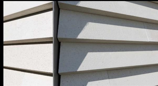
The technique of profiling in depressions and heights, in equal or different widths, also signals individuality on the basis of the matt terracotta surface. The effect on the surface can also be achieved by adding certain oxides, thereby creating irregular dots that stand out from the rest of the surface.
