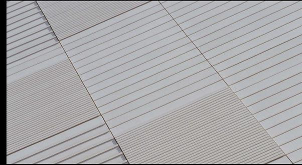
Structured TERRART® terracotta surfaces are increasingly being used in contemporary architecture as a design element in the form of natural, polished or peeled elements. Our range includes smooth ceramic surfaces that enhance the fineness of the material and numerous surface structures with different effects. This can influence both the look and feel of the ceramic facade.
