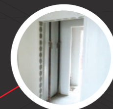
Internal walls and corridor openings
