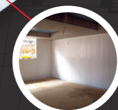
Basement and sub-basement walls
