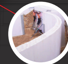
External façade and load-bearing walls
