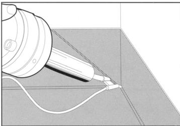
Use a hot-air gun for welding with thread at in-corners and out-corners. Tarkett Speed Welding Nozzle is specially designed for welding vinyl floors. For a perfect job, the Tarkett Swan Neck is required to effectively seal all seams nearest to the floor.
