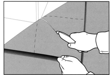
When fitting an out-corner, the sheet is folded against the corner and cut about 5 mm ( ¼ in.) from the floor. The guidelines in the picture show the corner on the sheet and the position of the cut at about a 45-degree angle. Then a diagonal cut is made as shown.
